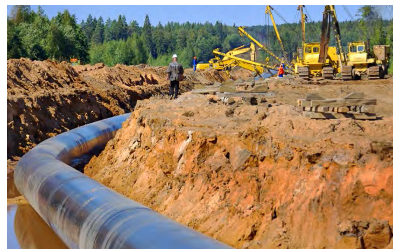
Construction of approximately 1000 kilometres of 48-inch diameter pipeline
