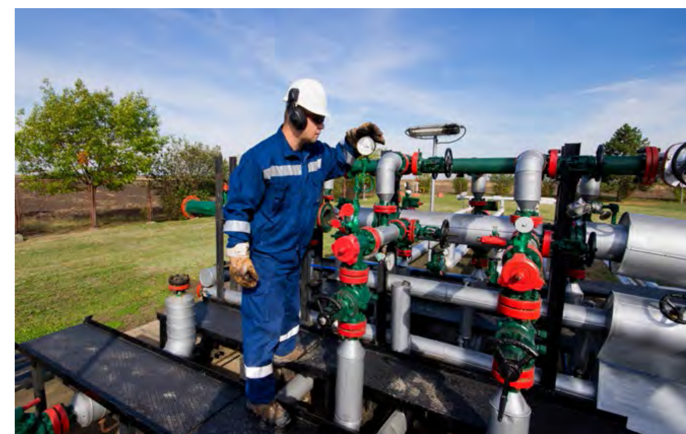
Construction and operation of metering facilities at the locations where suppliers provide natural gas to the pipeline and where natural gas is delivered to customers
